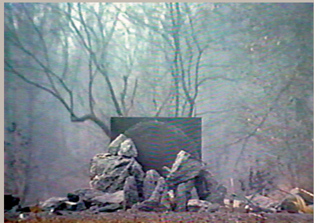
Remaining Rubble Can Be Removed
